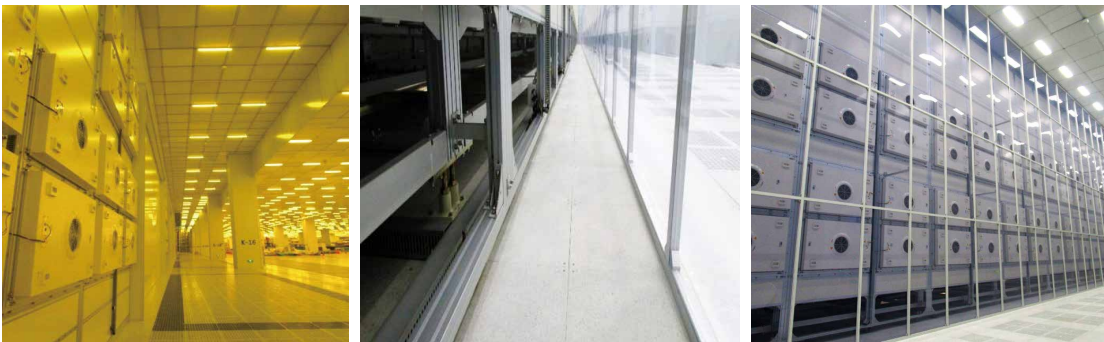
The on-site installation of the return vent filters
