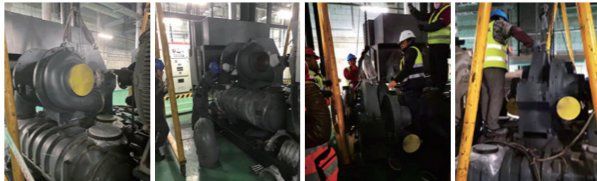
BOE Beijing Gen 5 TFT-LCD production line under CDA system renovation
