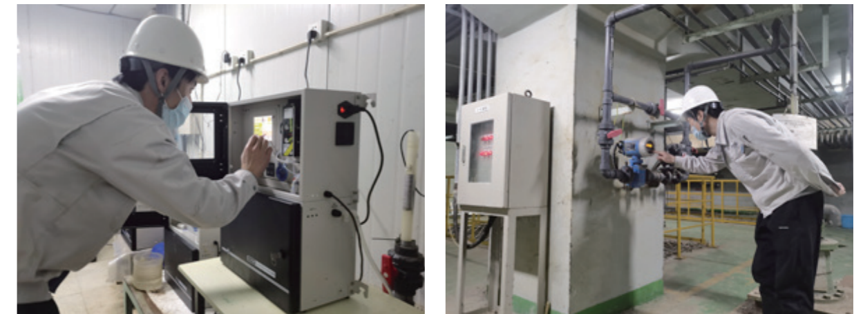
Employees check instrumentation and dosing systems
