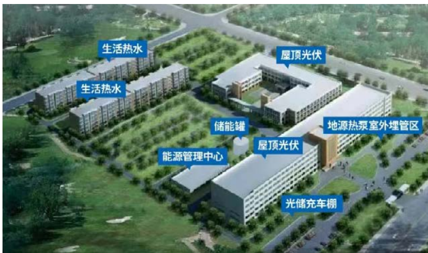
BOE's Near-zero-carbon Demonstration Park Project, with a 52% Energy-saving Rate and 37% Emissions Reduction Rate
