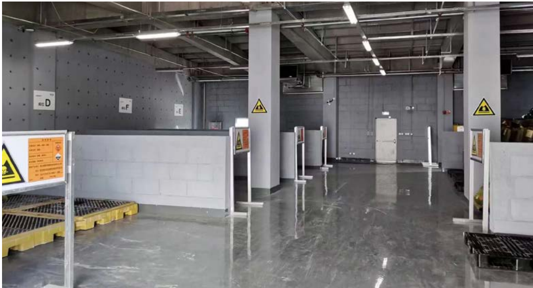
Hazardous Waste Storage at the BOE Ordos Gen 5.5 TFT-LCD Production Line
