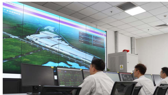
● Energy Management System
