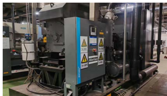
● Air Compressor Energy-Saving Retrofit
