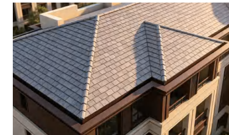
• Commercial residential building roofs
