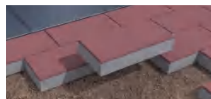
05 Laying surrounding materials
