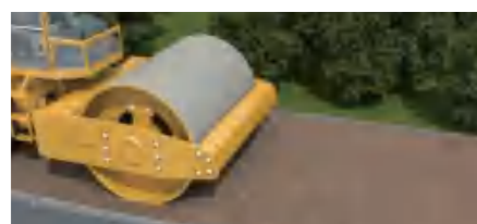
01 Ground base preparation
